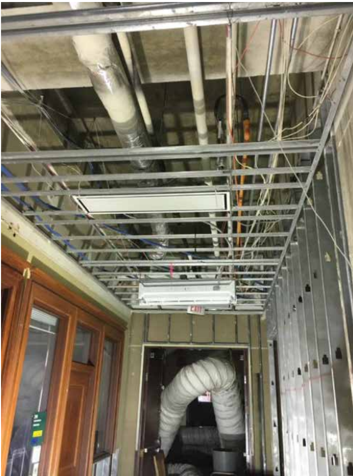
Second floor after ceiling tiles were removed.
