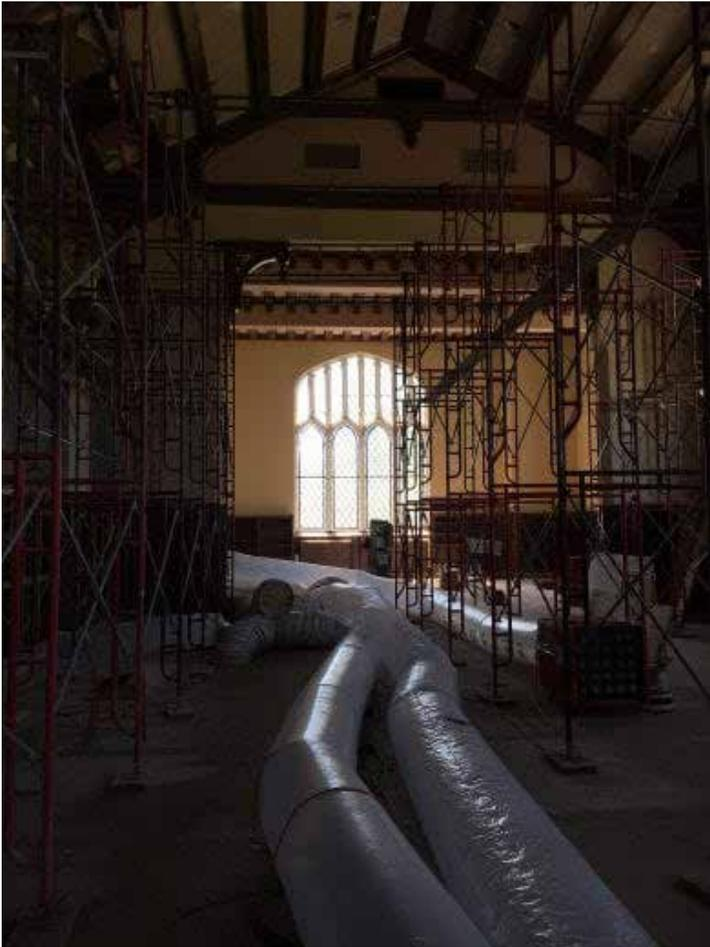
*The dehumidifier tubes removing moisture from the Great Room, and a second set of tubes is pumping chilled air in.*
