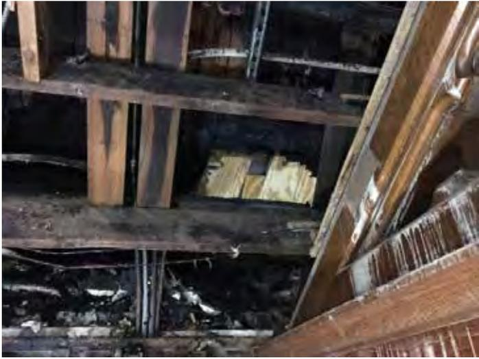
*Charred, scary holes up close and personal in the ceiling that have been covered by a temporary roof.*
