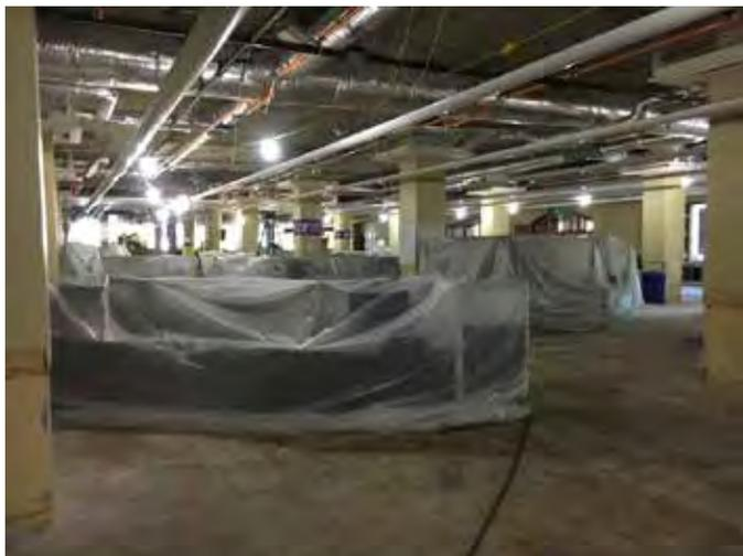
There was also extensive water damage to the drywall. In some areas, only a few feet needed to be removed, but in other parts, the entire wall had to be demolished and only metal studs remain.
