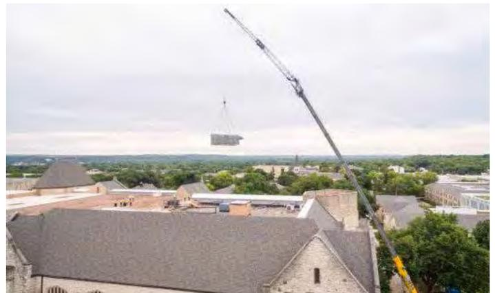
*Three massive heating, ventilation and air conditioning (HVAC) units on the roof that were close to the source of the fire were deemed not salvageable, so they had to be removed.*
