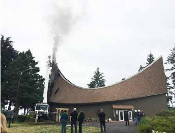
Demolition crews disassembled the roof structure. They preserved the original hardware and structural plates to be refinished and reused in preparation for the new, custom glulam beams.
