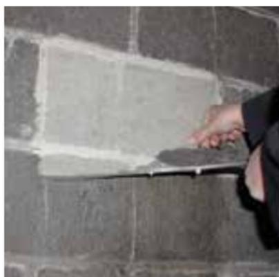
Surfaces such as concrete, brick, stone, plaster, dispersion paint, wood, plastic and metal that are dry or slightly affected will typically yield good results.
