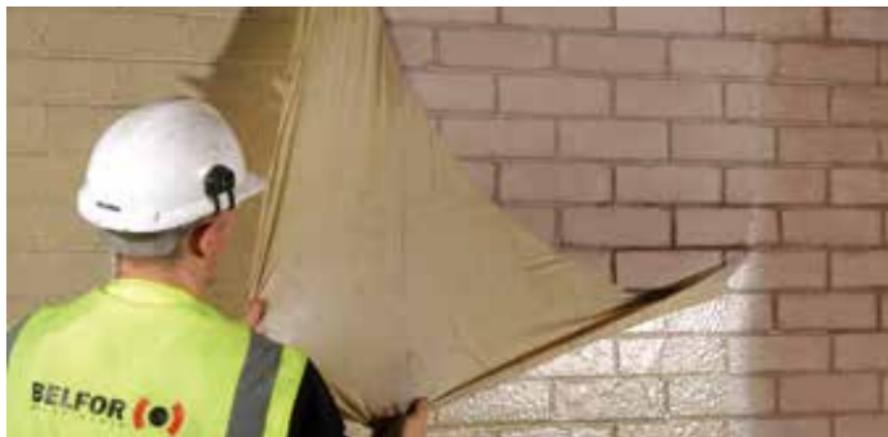
Dry film is removed — along with the soot, dust or other source of contamination — by pulling it off the affected surface.
