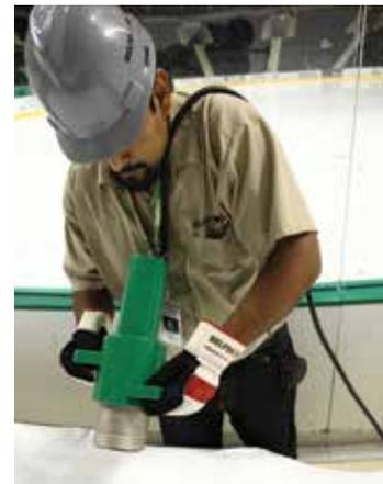
Although intended as a short term recovery solution, with proper care, maintenance and repair of tears/punctures, shrink wrap can extend the life of the temporary envelope for up to one year in some cases.
