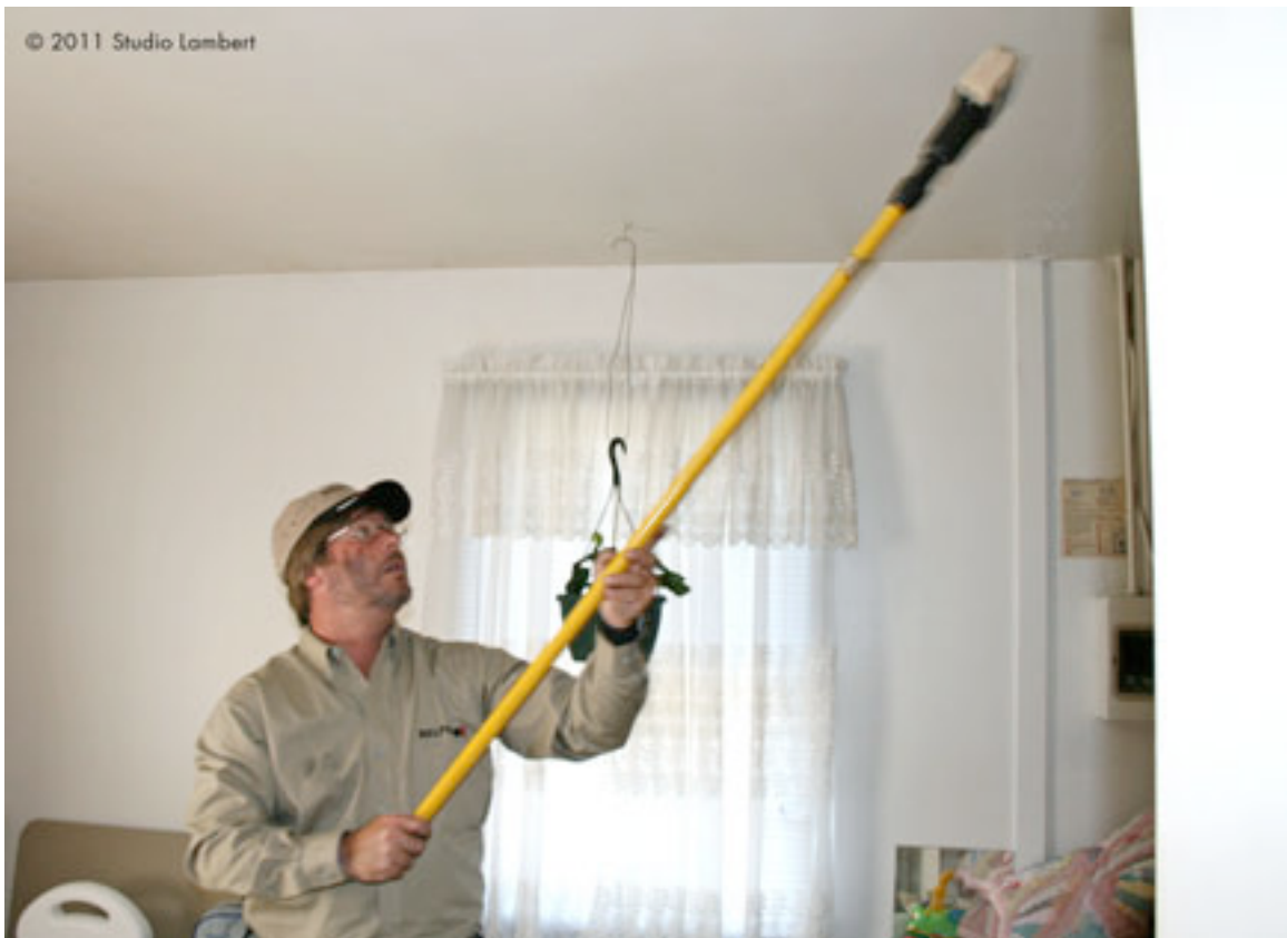
Sheldon works diligently to remove soot left in a home after a fire.
