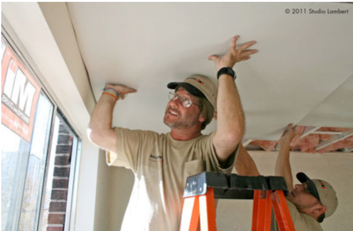
Drew lets Sheldon take the lead as they attempt to hang drywall together.
