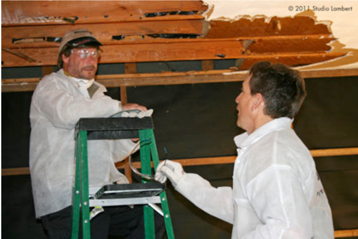
Joe and Sheldon hard at work repairing water damaged walls.
